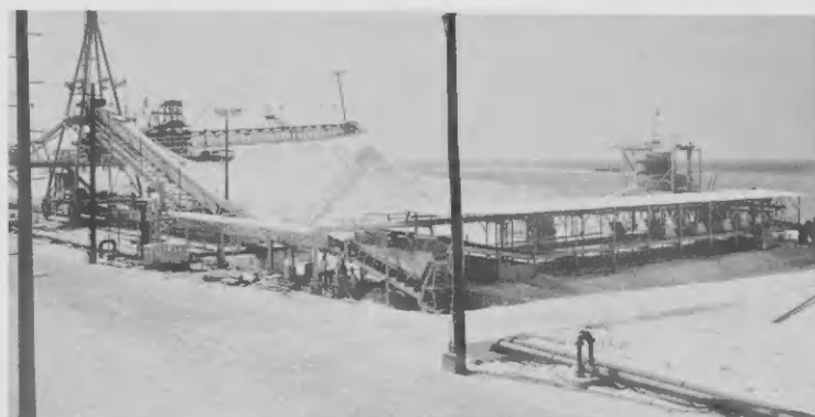
Lago's new sulfur handling facilities, with sulfur slaters in foreground and sulfur stacker to the left.
